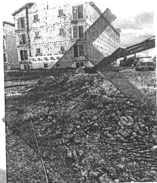
Figure 70 Parking lot excavation at building 8&9
