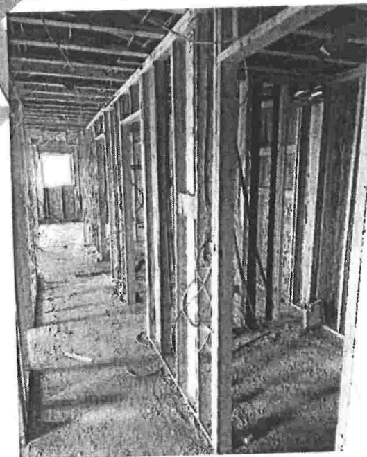
Figure 67 Building 10 Electrical Rough Ins
