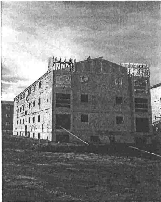
Figure 61 Building 11 Roof Framing
