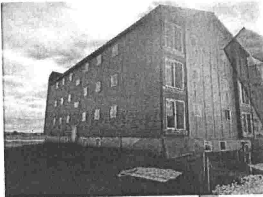
Figure 8 Building 1 - Northwest Elevation
