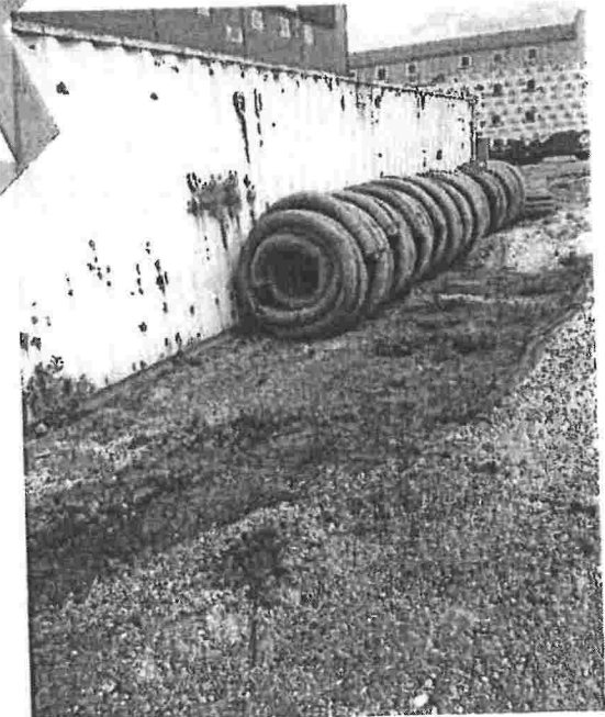
Figure 75 Weeping tiles on laydown
