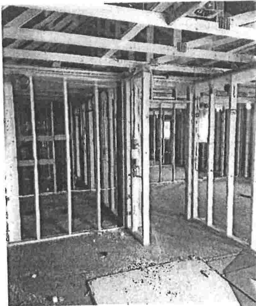
Figure 68 Building 11 Interior framing
