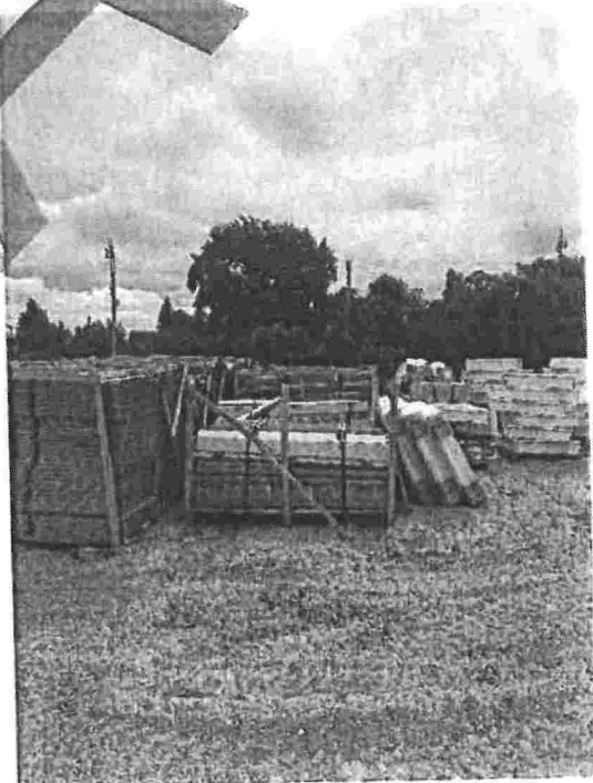
Figure 71 HM steel door and frame laydown
