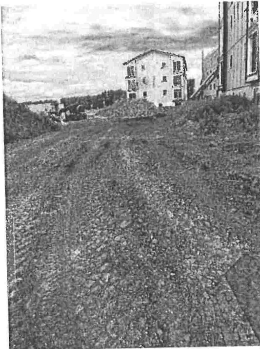
Figure 76 Parking lot on west grading
