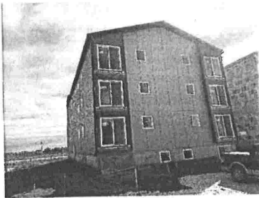
Figure 7 Building 1 -West Elevation
