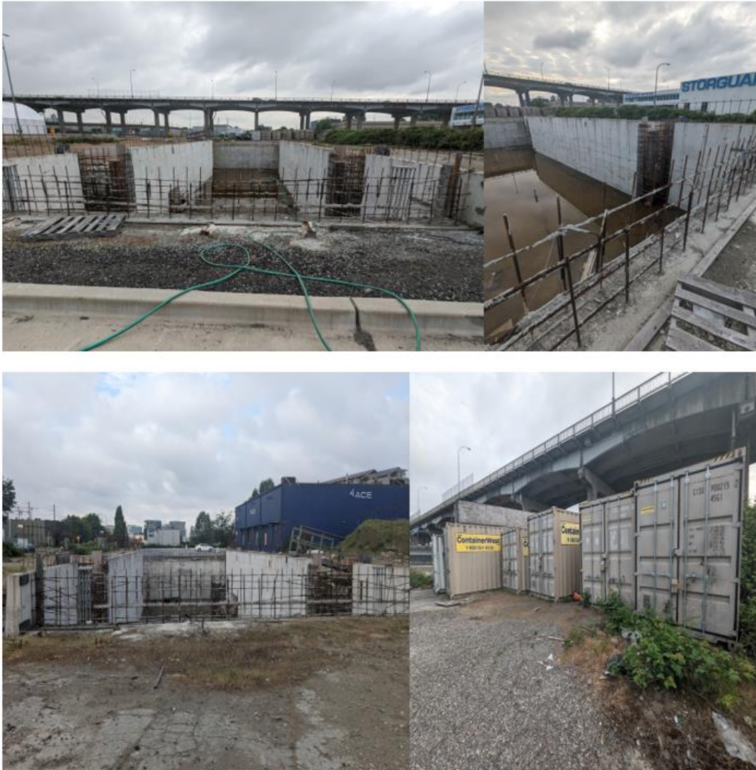
Images of development site and storage containers
