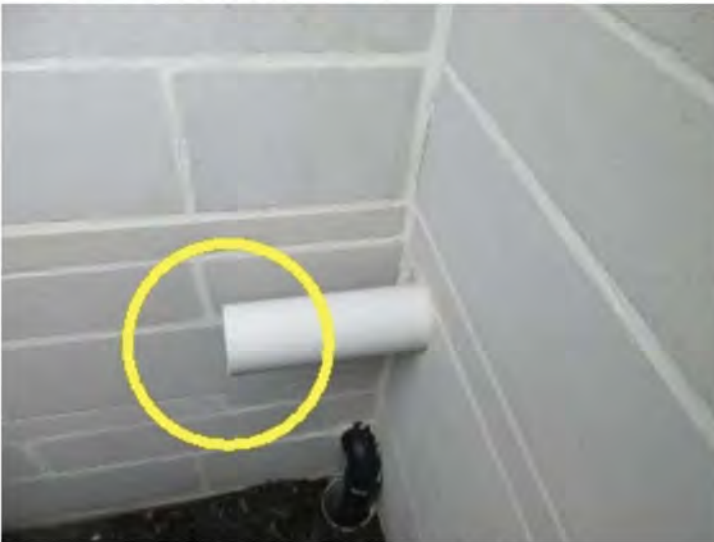
Scupper (flat roof drain)
