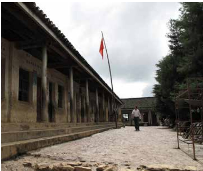
Yunnan Hope School: The school building – before and after
