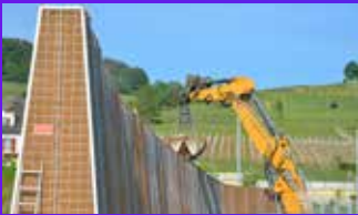
Reservoir tsunami protection barrier, Tyrol, Austria
