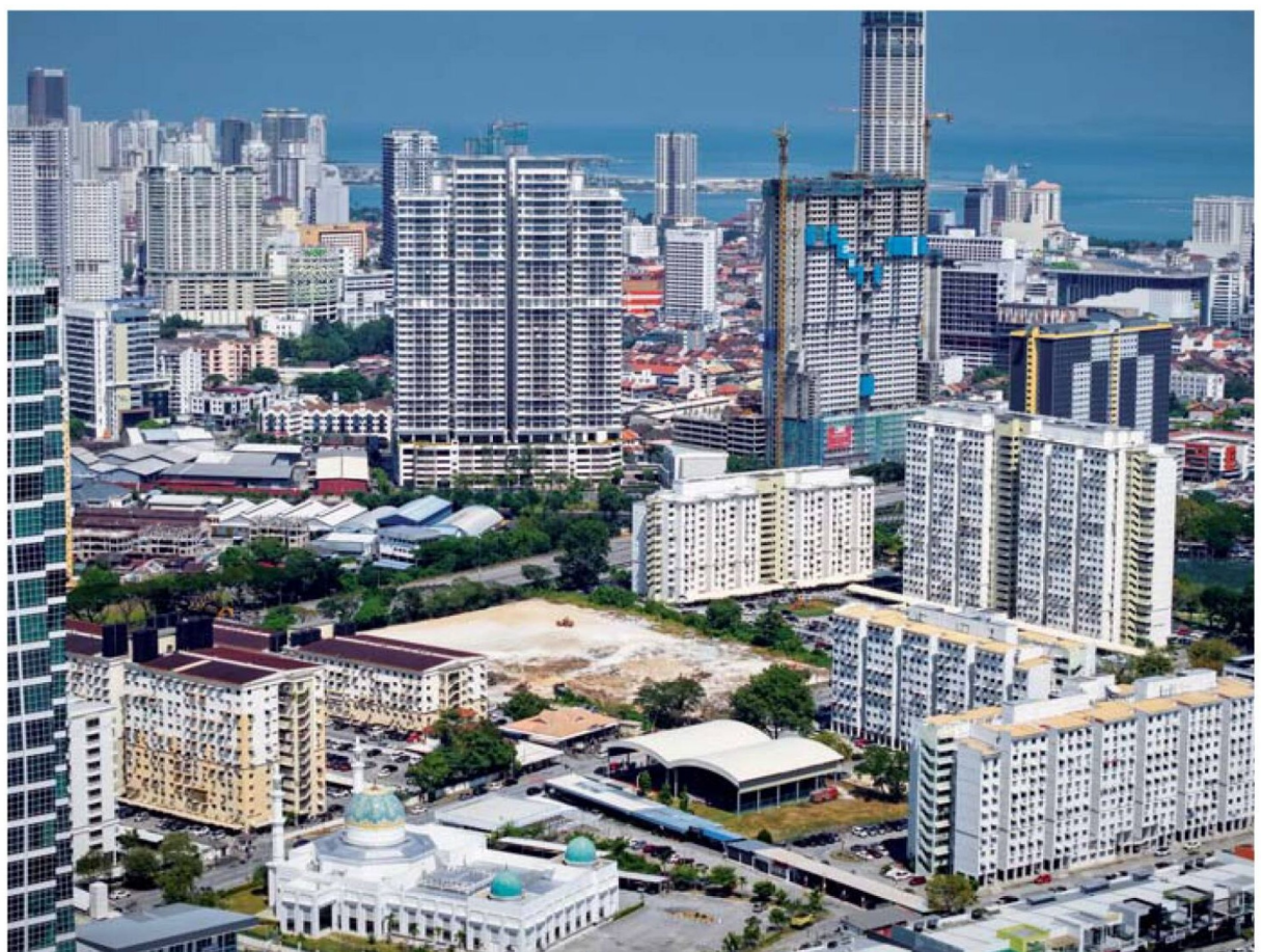
The site of the upcoming Bandar Seri Pinang LRT station site in George Town
