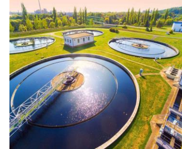
Water / Waste Management
