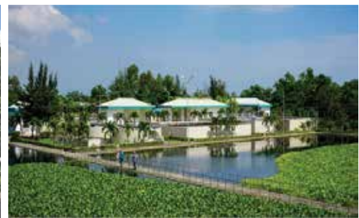
Centralized waste water treatment plant in Dien Nam-Dien Ngoc IZ
