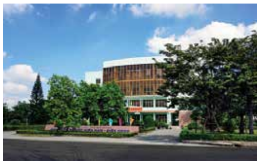
Operation building of Dien Nam – Dien Ngoc IZ
